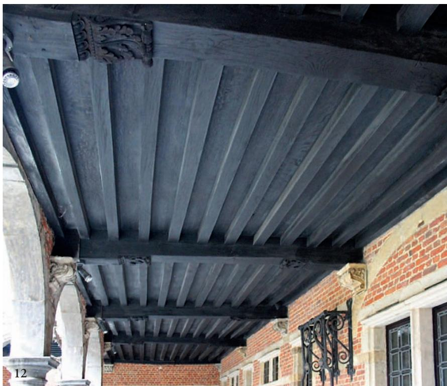
4 Gravensteen Castle, under chamber, ties set directly in masonry. Wall pockets evidence of earlier ceiling.
